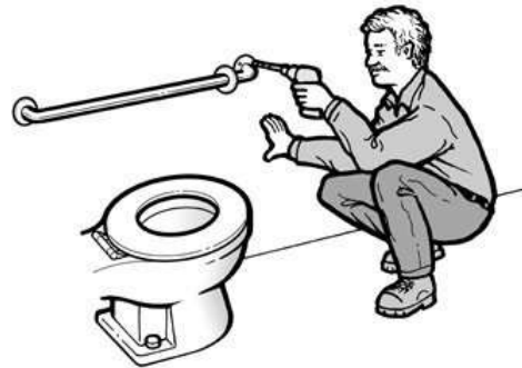
Grab Bar Installation
