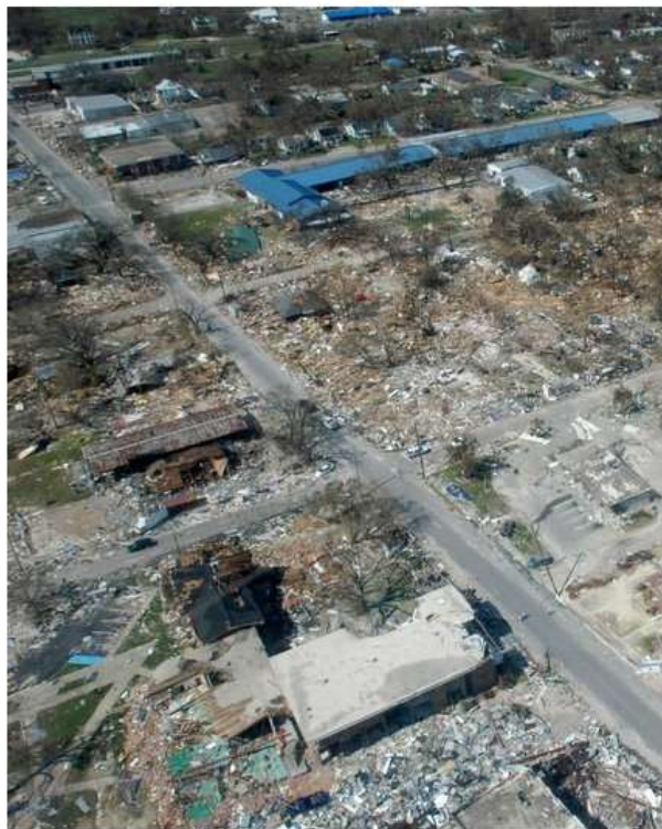
Hurricane Katrina Damage: Gulfport, Mississippi 2005
